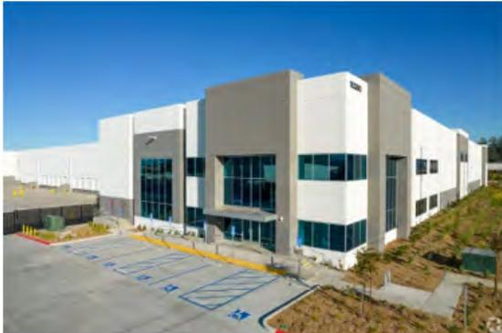
Typical Building Design with Concrete Wall Panels
